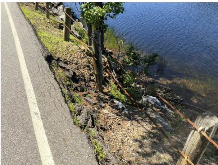
Eroding roadside down a steep bank (top left, top right, bottom left) leading to sediment deposition into Lake Winona (right).
