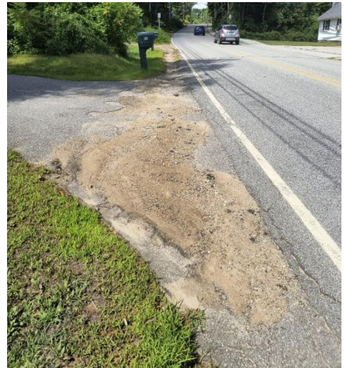
Erosion of house #98 driveway (left) that travels down the road, gullying the ditch (middle) and erodes and deposits sediment on the driveway of house #96 (right).
