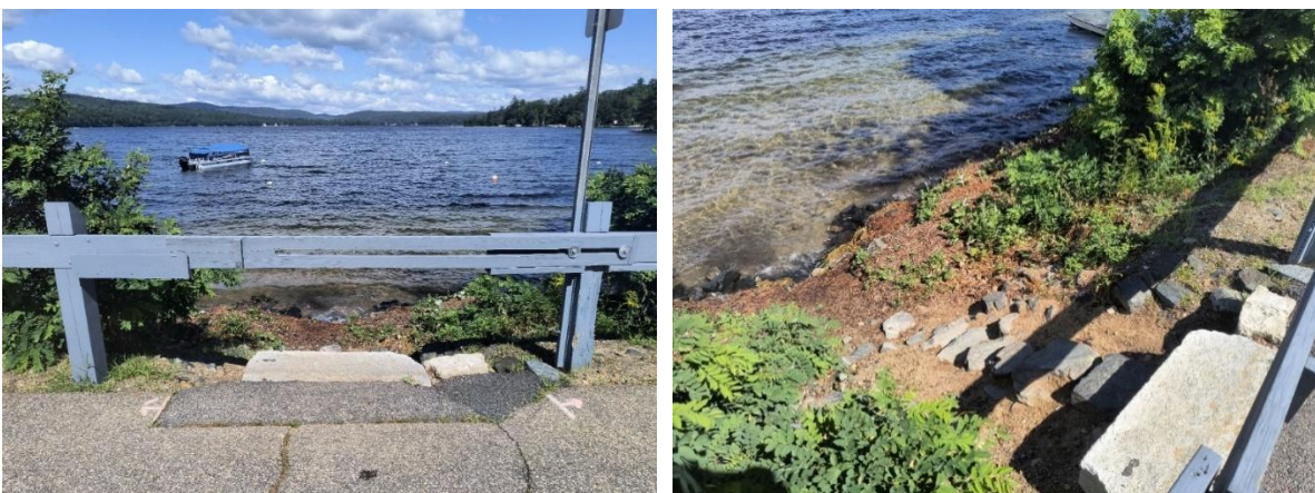
Launch gate from road (left) and steps for launch to water (right).
