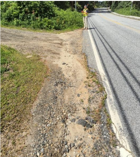
Erosion of house #98 driveway (left) that travels down the road, gullying the ditch (middle) and erodes and deposits sediment on the driveway of house #96 (right).
