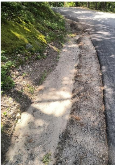
A gully full of sediment (left) leads to catch basin (middle). Road intersection island with catch basin in roadway (right).
