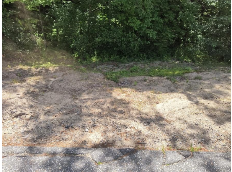
Road shoulder erosion and sediment deposition on Piper Hill Road (left and right).
