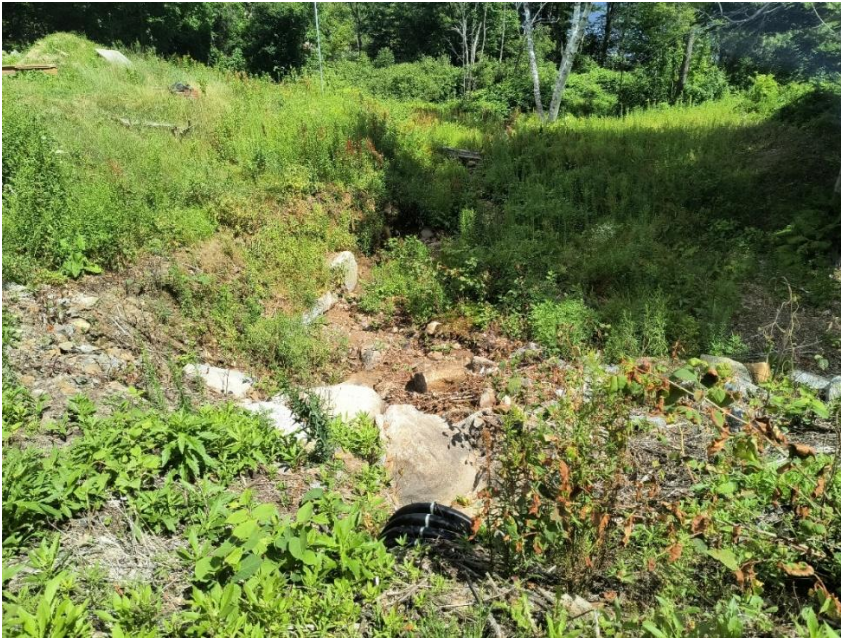
Road shoulder/ditch erosion and sediment transport (left and right).
