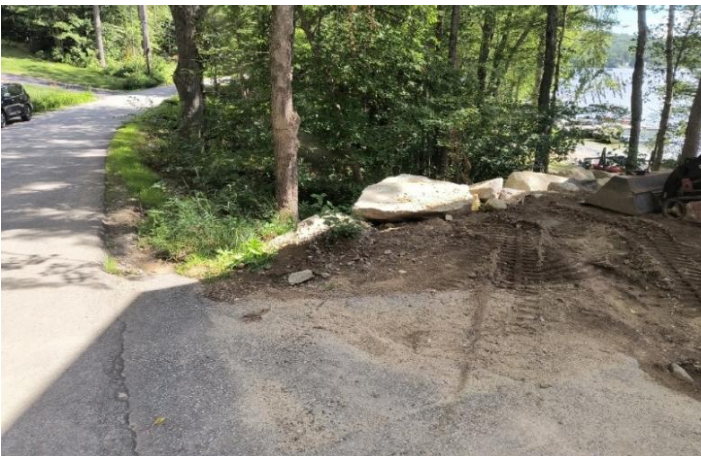
New construction (left) with stream on other side of rock wall and small silt sock. Some visible gully on side of road (right).
