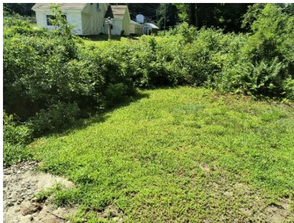
Road shoulder erosion and sediment transport straight to culvert (left and middle). Area where a rain garden could be planted to divert stormwater to (right).
