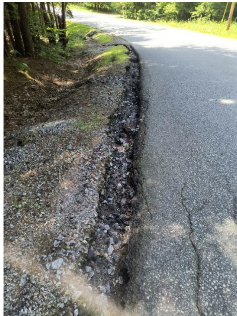
Stormwater forms a gully along the road shoulder that deepens (left and middle) until it travels into the road ditch through several gullies (right).
