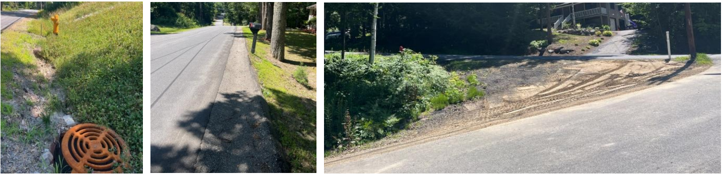
Catch basin to underground drainage system (left). Paved swale (middle). Loose dirt on corner for DPW material staging (right).
