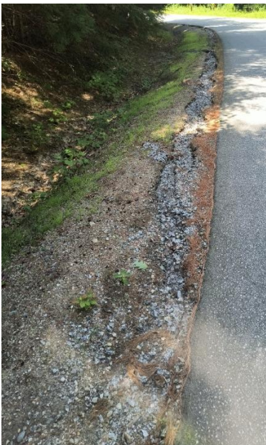
Stormwater forms a gully along the road shoulder that deepens (left and middle) until it travels into the road ditch through several gullies (right).
