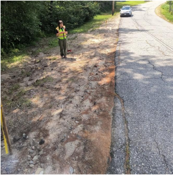
Road shoulder erosion and sediment deposition on Piper Hill Road (left and right).
