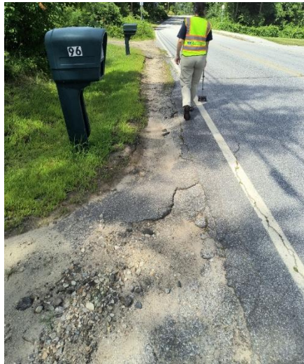
Erosion of house #98 driveway (left) that travels down the road, gullying the ditch (middle) and erodes and deposits sediment on the driveway of house #96 (right).
