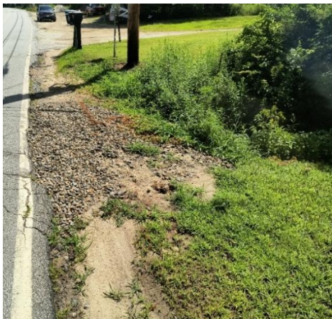
Road shoulder erosion and sediment transport straight to culvert (left and middle). Area where a rain garden could be planted to divert stormwater to (right).
