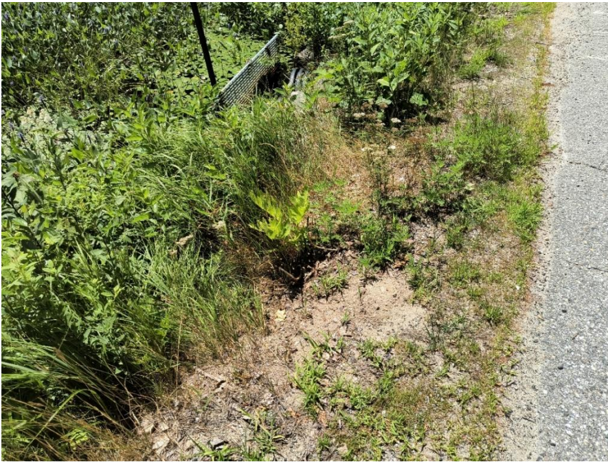
Edge of road and wetland with lack of buffer (left). Eroding road shoulder with ample sediment buildup (right).
