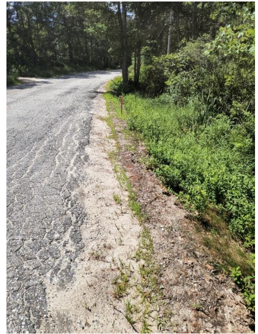
Edge of road and wetland with lack of buffer (left). Eroding road shoulder with ample sediment buildup (right).
