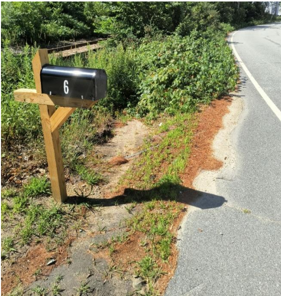
Slight sediment transport to ditch (left) and sediment build-up on road surface (right).
