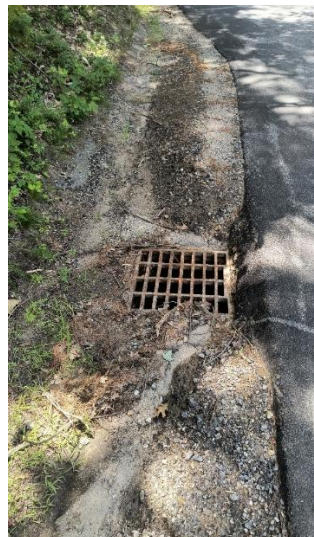
A gully full of sediment (left) leads to catch basin (middle). Road intersection island with catch basin in roadway (right).
