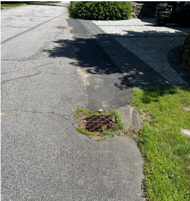
Catch basin in the middle of pavement (left) and the stream to which it discharges (right).
