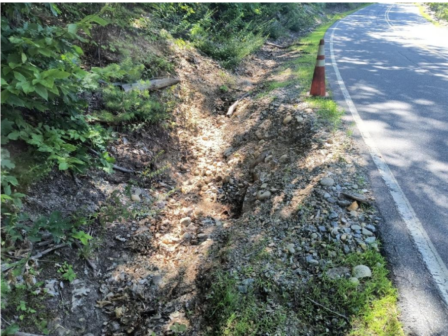
Eroded culvert inlet and road shoulder (left) transporting sediment and organic material through to the outlet and lake (right).
