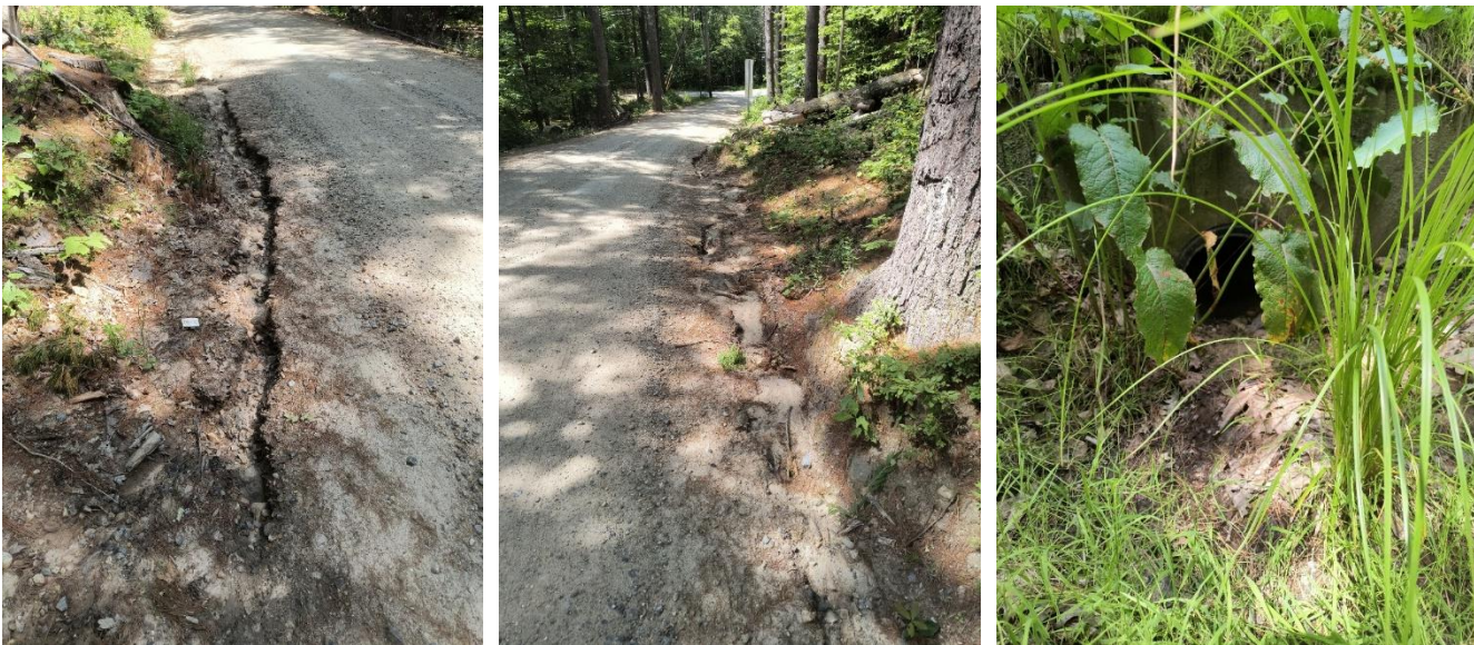
Gully along roadside (left and middle) that drains to culvert (right).
