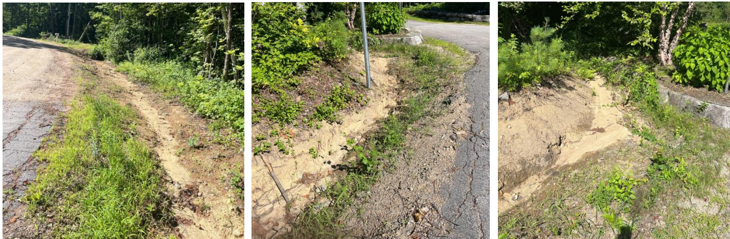
A gully in the road ditch (left) leads to an intersection (middle) and outlets into the woods (right).
