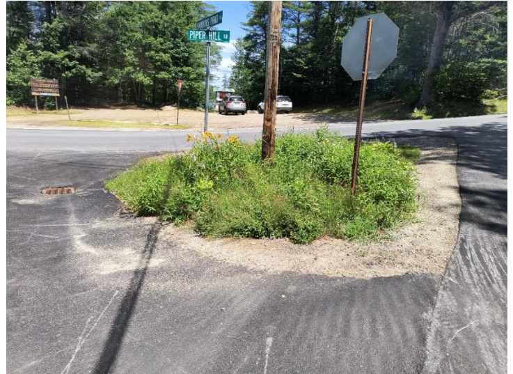
A gully full of sediment (left) leads to catch basin (middle). Road intersection island with catch basin in roadway (right).
