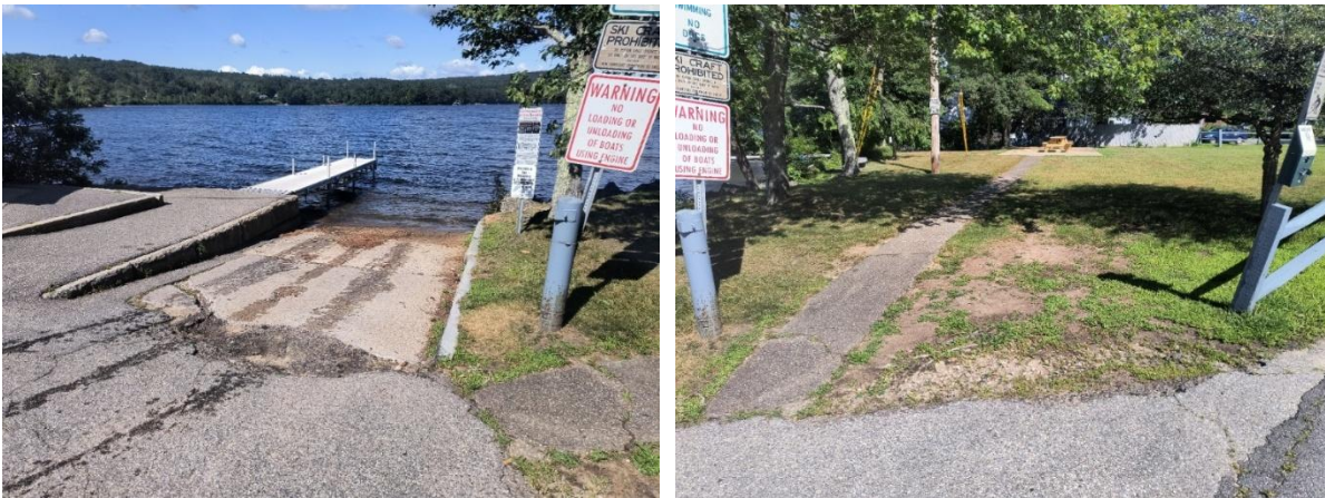
Boat ramp (left) and adjacent park (right).
