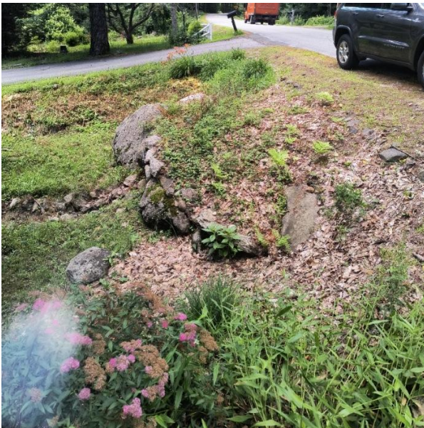
Culvert inlet with minimal vegetation.
