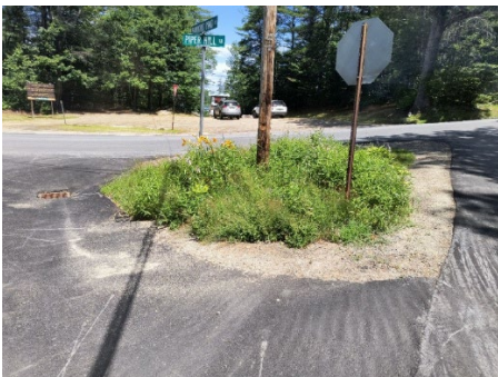
A gully full of sediment leads to a catch basin (top). Road intersection island with catch basin in roadway (bottom).
