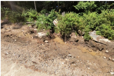
Washed out check dams caused gullies to form in the road ditch.
