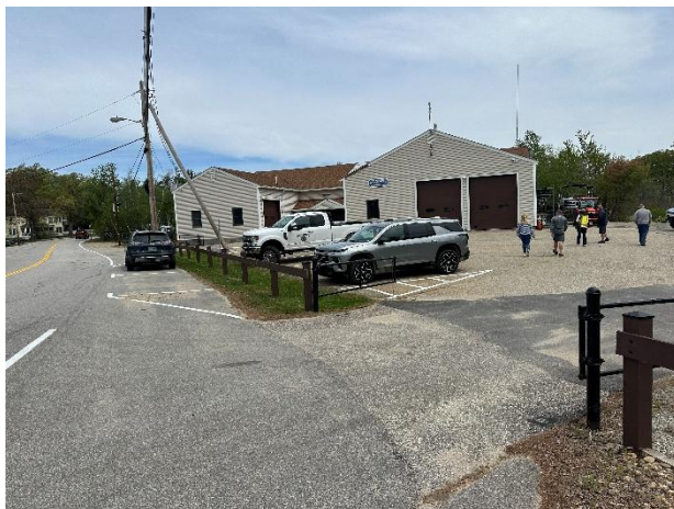
Photo 15: Meredith Water Department water treatment facility.
