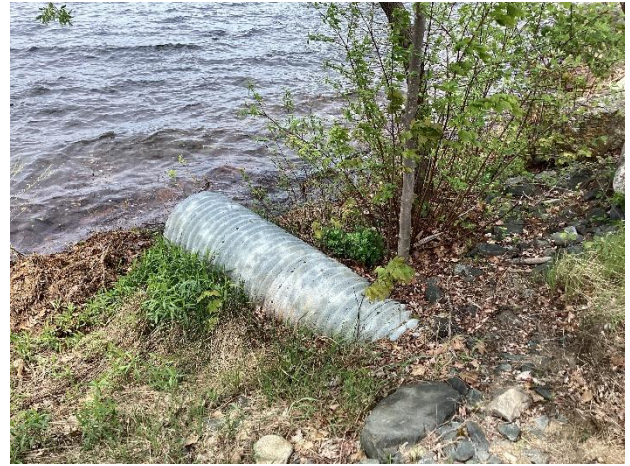
Photo 12: Corrugated metal outfall pipe near concrete steps south of the boat ramp.
