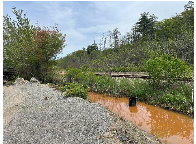
Photo 16: Ditch along railroad track to the south of Water Department building and drive.
