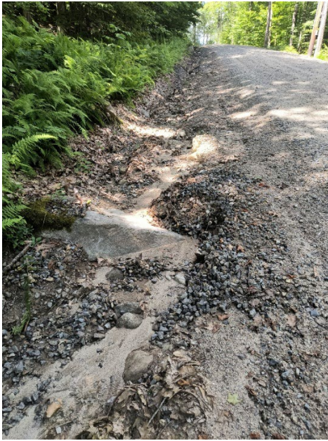
Washed out check dams caused gullies to form in the road ditch.
