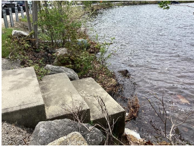
Photo 11: Corrugated metal outfall pipe near concrete steps south of the boat ramp.
