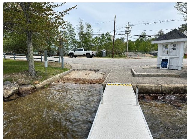
Photo 2: Boat ramp and dock, facing east.
