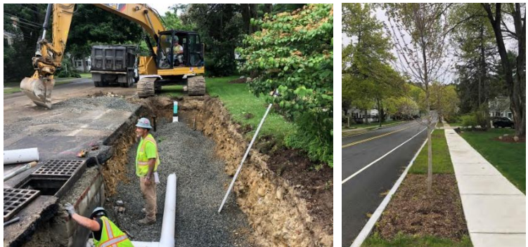
Example stormwater tree trench
